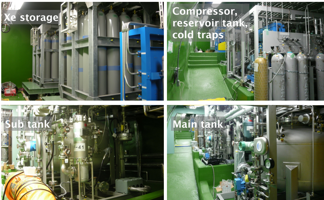
Figure 3.22: A schematic view of Xe handling system and each picture.
