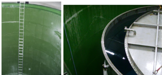
FIG. 5: The feature of the veto tank(left) and the buffer tank filled with water(right).
